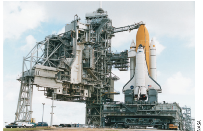
FIGURE 1-4 Space shuttle being made ready for its launch into space. Notice the large welded support structure used to prepare the shuttle for launch.
